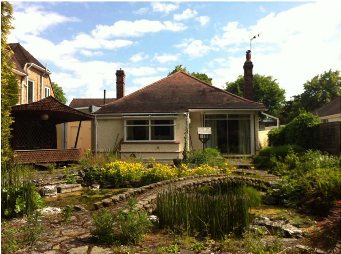
Photo 2. 27 Private Road (rear)
